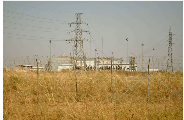
An oil installation in Sudan. Image credit: Shannon Orcutt/SaveDarfur/Flickr
