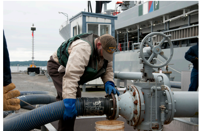
Loading a 50/50 biofuel and petroleum blend aboard the oiler, USNS Henry J. Kaiser
