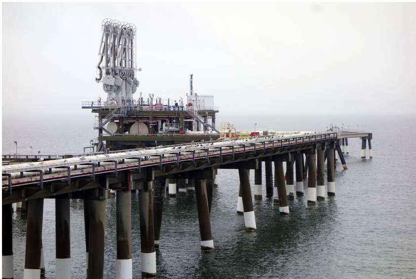
The pier at Dominion's Cove Point liquefied natural gas (LNG) plant on Maryland's Chesapeake Bay in 2014. PHOTO: TIMOTHY GARDNER/REUTERS
